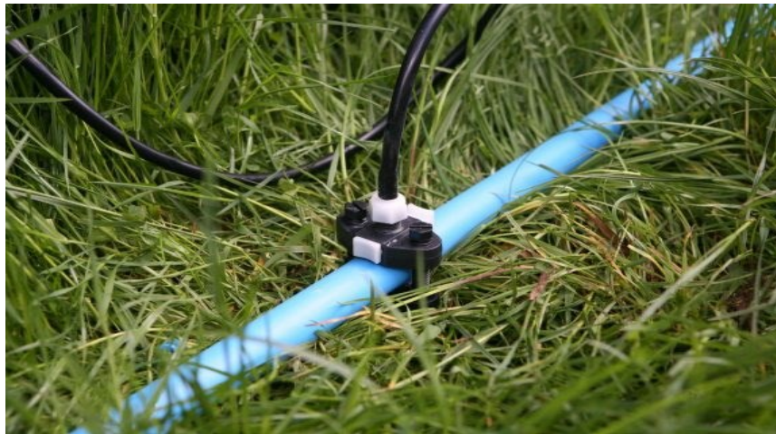
SADDLE CONNECTOR CLAMPED TO ALKATHENE PIPE AND BLACK TUBING FITTED.
